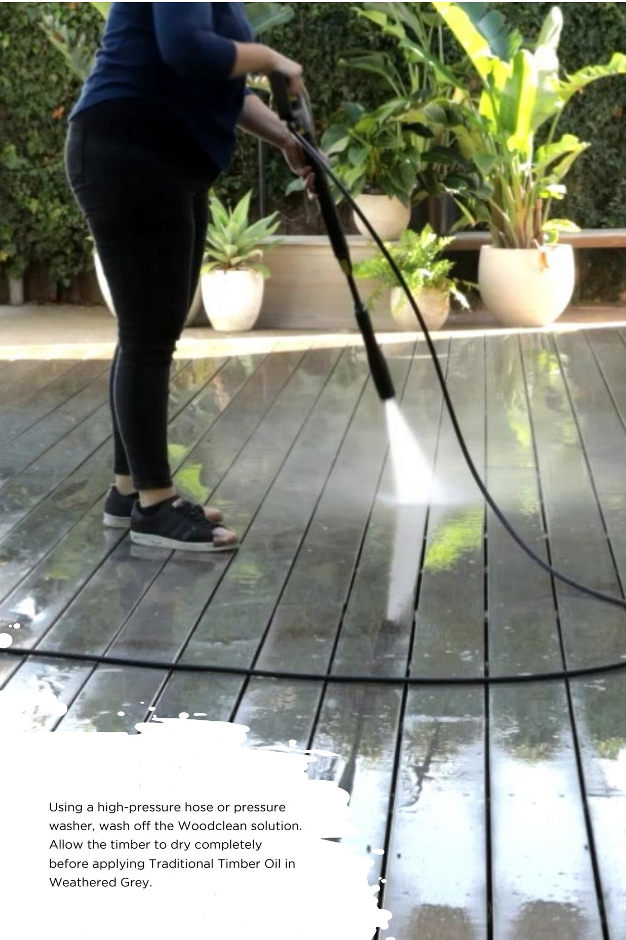
Using a high-pressure hose or pressure washer, wash off the Woodclean solution. Allow the timber to dry completely before applying Traditional Timber Oil in Weathered Grey.
